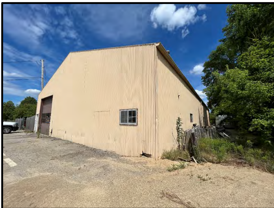
SUBJECT BUILDING – FACING NORTHEAST
