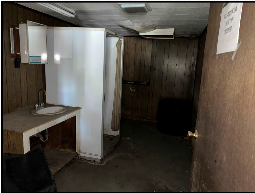
SUBJECT BUILDING INTERIOR BATHROOM
