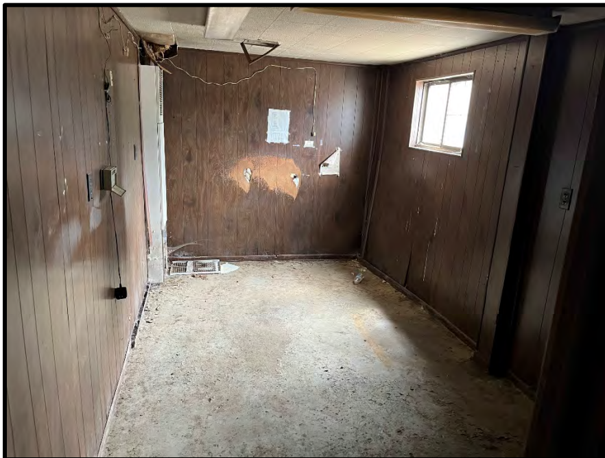
SUBJECT BUILDING INTERIOR OFFICE AREA
