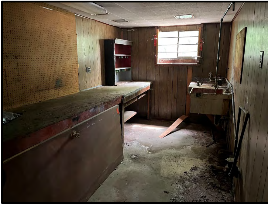
SUBJECT BUILDING INTERIOR STORAGE ROOM
