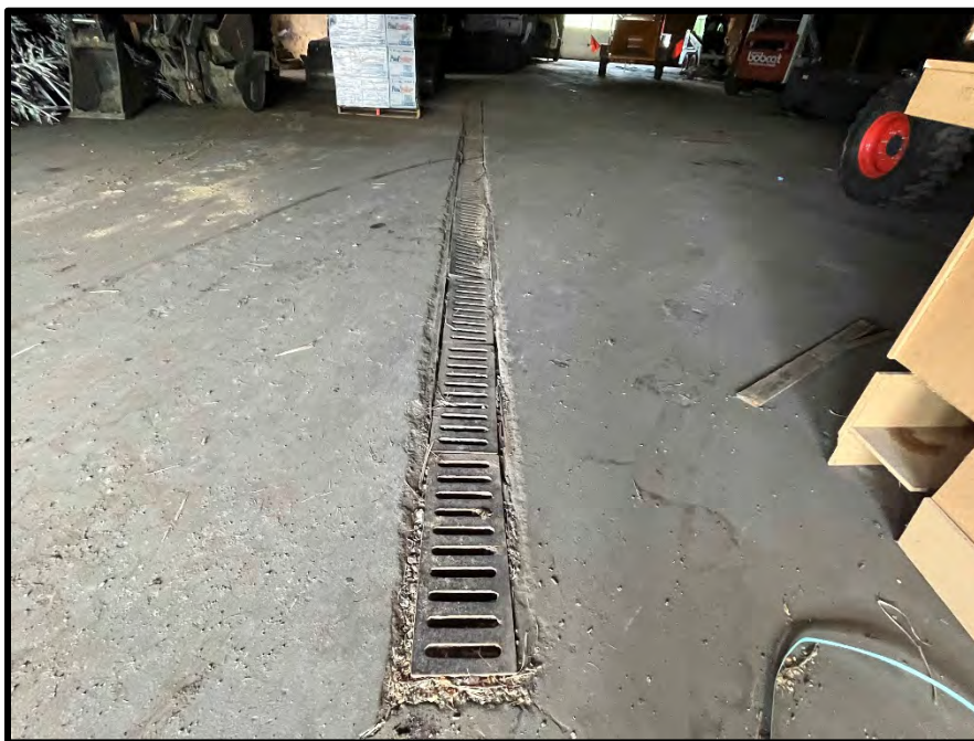
VIEW OF TRENCH DRAIN LOCATED IN THE WESTERN PORTION OF SUBJECT BUILDING
